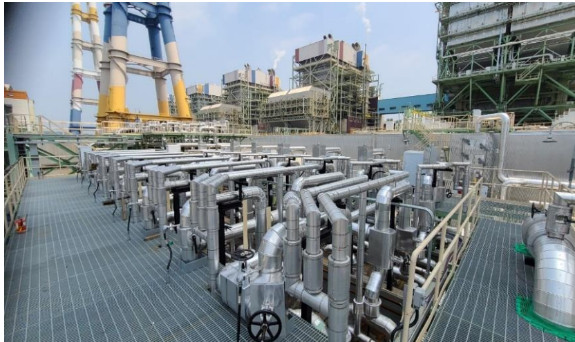
<#5,6 GGH, Absorber, UREA, Limestone, etc. piping>
