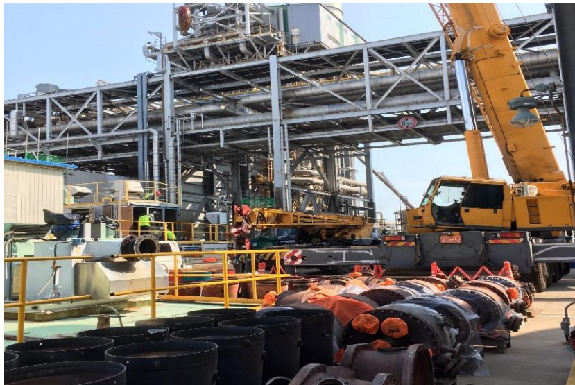
<GT 3&4 disassembly and inspection>
