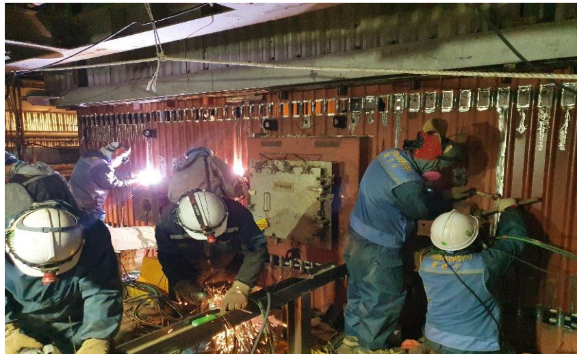
<SH Replacement and Wall Panel Replacement>
